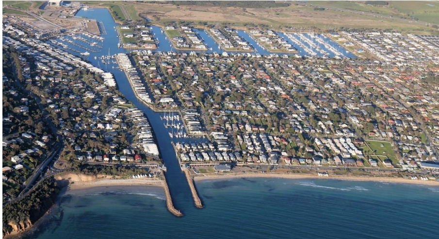
Figure 3 Entrance of Martha Cove Marina, formerly Brokil Creek, showing breakwaters which 'train' the entrance to maintain its location and dimensions (Neville Rosengren, June 2019)
